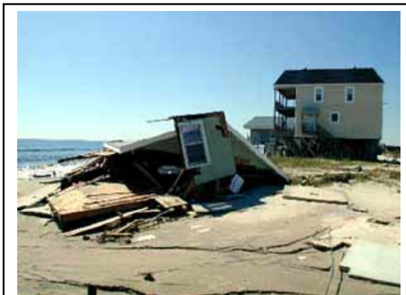
Hurricane Floyd brought a devastating 15 feet of storm surge that damaged or destroyed hundreds of houses along the ocean front of Long Beach on Oak Island, North Carolina in September 1999. A prime example of successful hazard mitigation, the elevated home (right) survived while the older, ground-level block foundation of the home on the left was undermined and crushed. (Photo by Dave Gatley/FEMA News Photo)
